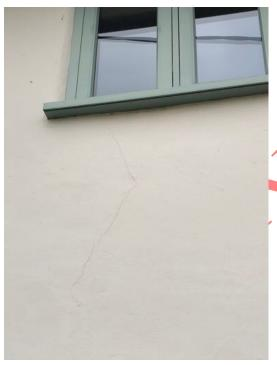
Informative: clay lump buildings require lime or earth based renders and special treatment when redecorating render / impervious coatings. Modern cementifitious renders and modern paint are not usually appropriate, and use of such may cause damage to the underlying wall structure. You should ensure that any contractor you instruct is experienced in this building type.
