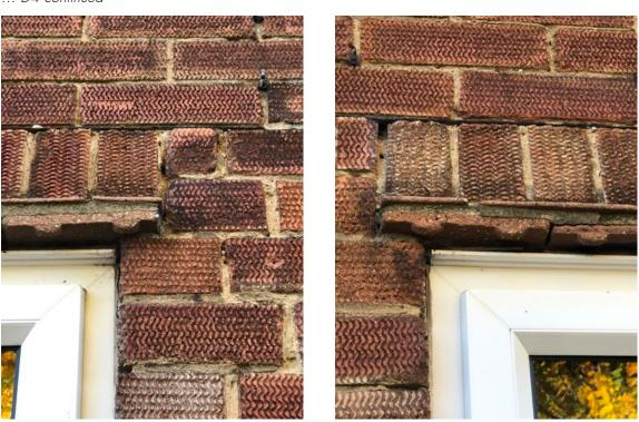
Airbricks provide ventilation to the subfloor void, and you should ensure these are kept clear to maintain airflow and prevent condensation in the subfloor void. Condition Rating 1.
