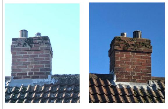
Informative: Chimney stacks are particularly exposed to the weather and so regular maintenance must be carried out to ensure their stability and weather tightness
