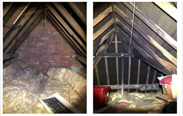
Informative: any items stored in the roof should be of lightweight nature and spread evenly in the roof void to avoid the possibility of damage to the ceilings thereunder. Rafter/purlin construction was not designed to allow for excess weight and therefore the storage of items is discouraged.
